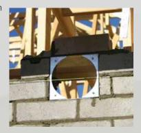
The outlet includes generous space for the attachment of ducting and has been optimised to suit two standard courses of standard 76mm bricks.
