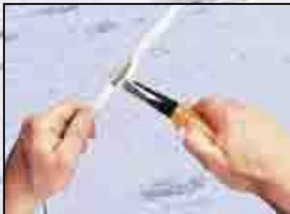
1. Remove outer sheathing only to required length.
