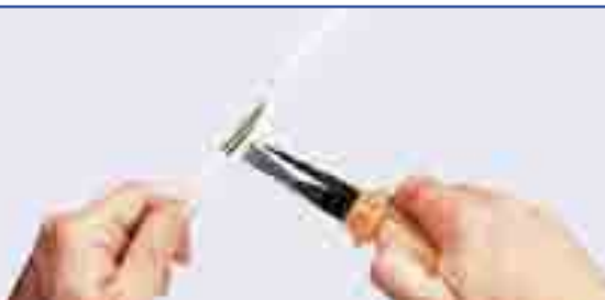
1. Remove Outer Sheathing of TPS Cable (46mm - Mid Connection or 70mm - End Connection)
