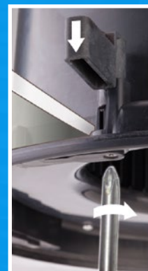
Tighten screws so clips clamp onto ceiling board.
